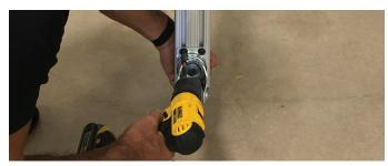
**9.** Install casters on to bases using the 16 hex head screws and 16 rail nuts.
