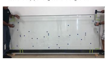
**3.** Lay the 10' single rail on wooden blocks and place glass in rail slot, centered. Glass should protrude 1/4" on each end of rail. Use mallet to seat glass in the rail.
