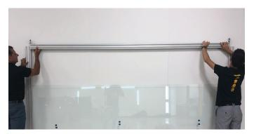
6. Slide the 10' double rail down the 2 upright rails to the glass. Use mallet to seat the rail on the glass if needed. Then tighten screws to uprights. At this point all fasteners should be tight and glass should be seated on all 4 sides. Cut tape at gasket and remove excess tape.
