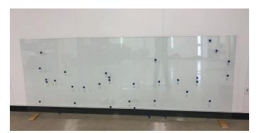
**1.** Stand 4' x 10' glass up on the 10' edge. Place on wooden block spacers. Place one on each end. Measure and cut gaskets, Cut (2) 3' long sections & (2) 9' long sections of gaskets.
