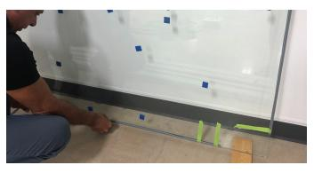
**2.** Install glass gaskets on all 4 edges of glass. Place 3' gasket section on the 4' edges and 9' gasket on 10' edges. Using masking tape, tape center and ends of gaskets to hold in place.
