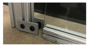
**4.** Fasten two 3" flat brackets on the end of each 6' double rail and attach to the 10' single rail on the floor. Use mallet to seat rails on to the glass if needed.
